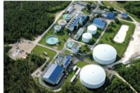
FKAA J. Robert Dean Water Treatment Plant in Miami Dade County
