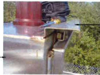
DRIPSHIELD/RAINGUARD DETAIL
