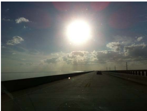
7-Mile Bridge south of Marathon
