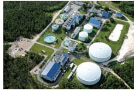
FCAA J. Robert Dean Water Treatment Plant in Miami Dade County
