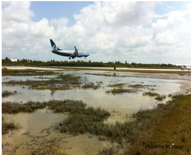
Key West Airport flooding effects solely from high tide in May, 2012
