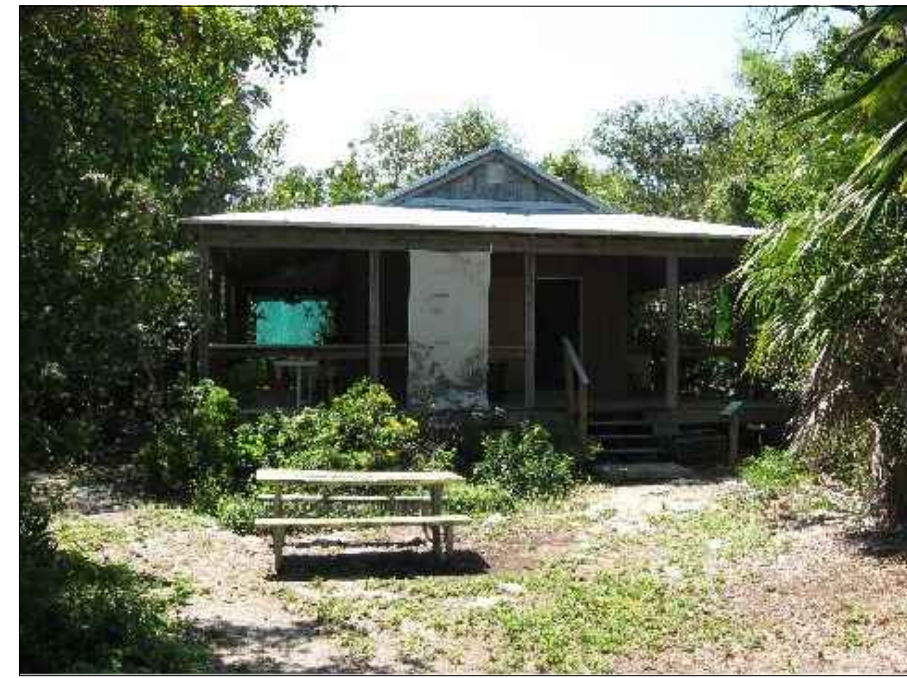
CRACKER HOUSE START
